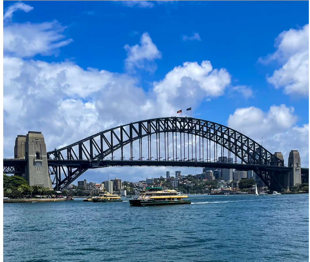
Sydney Harbour Bridge
